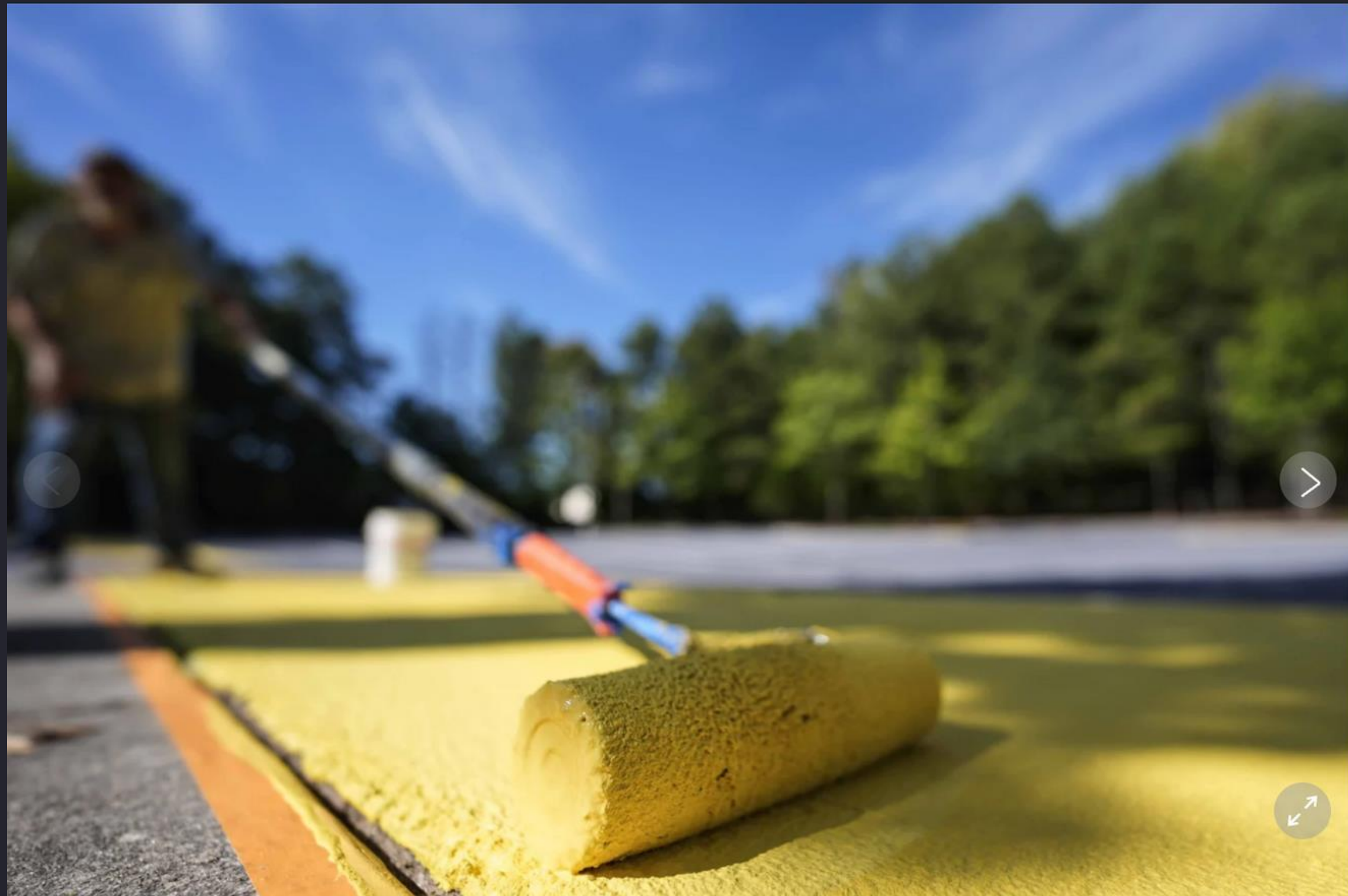
1 of 4 | Ronnie Jefferies paints the parking lot at Science, Arts and Entrepreneurship School to help cool it by making it more reflective, Wednesday, Sept. 4, 2024, in Mableton, Ga. (AP Photo/Mike Stewart) Read More
