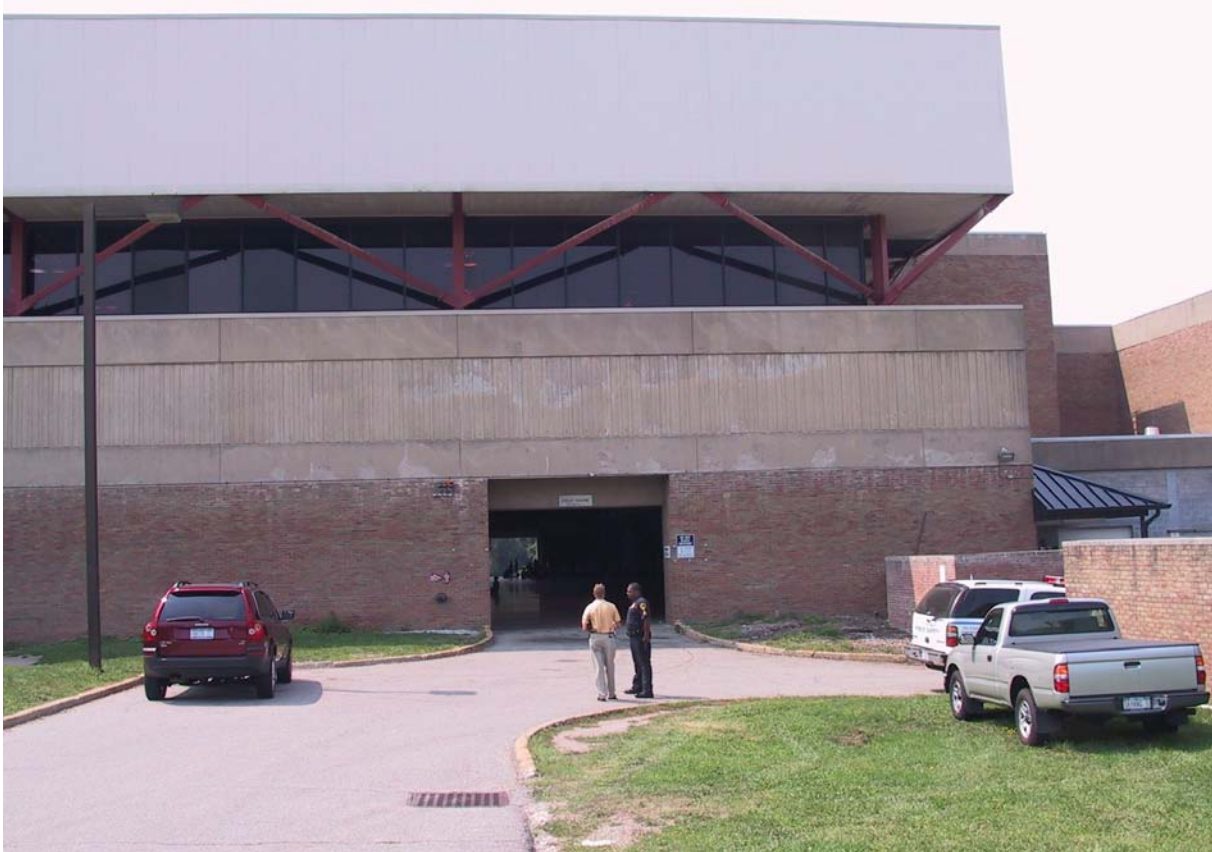
Photo 1. The Field House entrance where the aerial work platform was parked during the incident.
