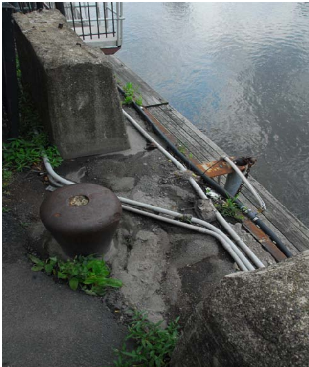
Photo 1. The area where the victim fell. The floating docks shown here were placed in the water after the incident.
