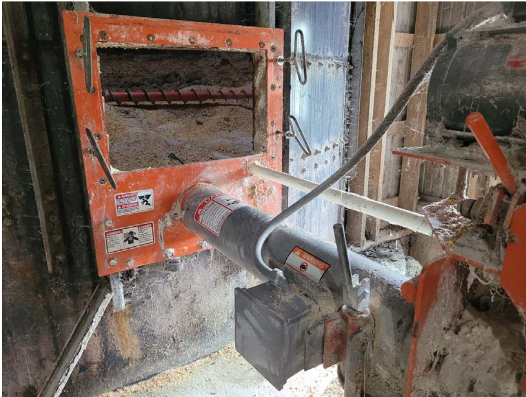
Photo 6. Access door in the base of the silo.
