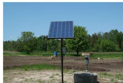
**Simple Pump installed in an old pit well provides water to the community garden in Clay, New York. (Photo credit: SunshineWorks.com)<sup>111</sup>**
